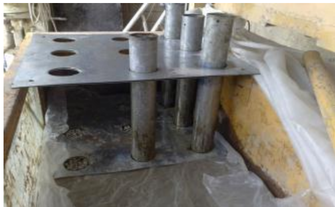
Plate 7. The process of stone column installation.
