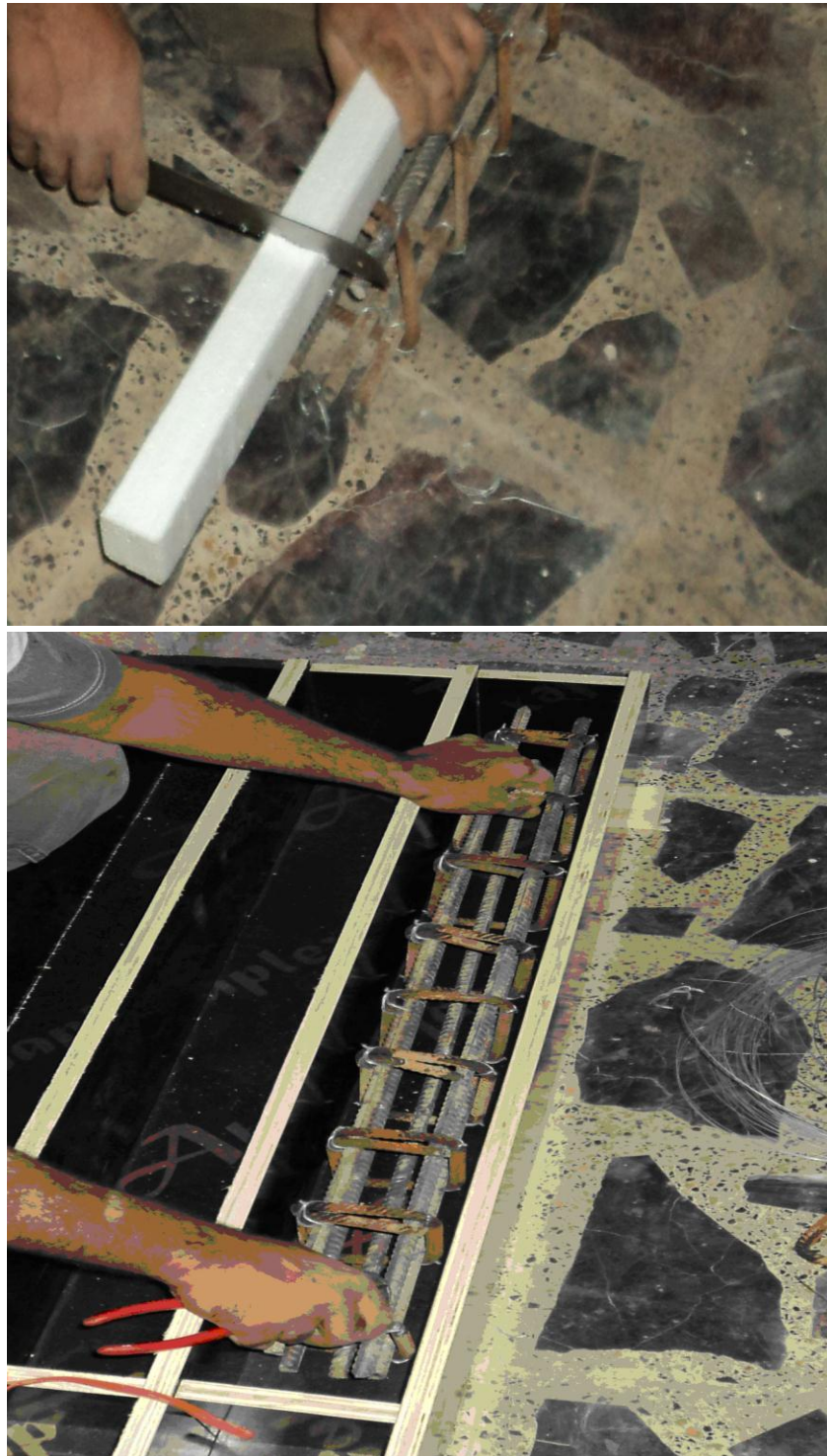
Figure 1. Moulds of reinforced concrete solid and hollow reinforced concrete beams.
